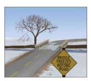
The bridge would become icy first because it loses heat over its entire surface. The bridge would lose heat by radiation, conduction and convection to the colder air from its top, sides and underside. The net result is that the bridge's surface temperature would closely trend the air temperature.
